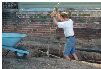
Jul 14 Jim Roepke, Master Stone Mason, digs the foundation
